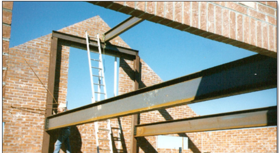
Steel beams allowing greater headroom.
