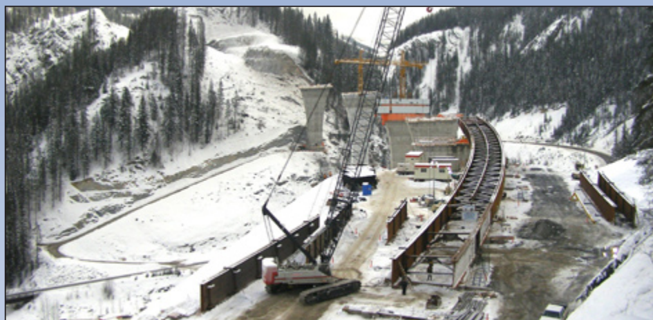
Two girder assemblies before launch.
