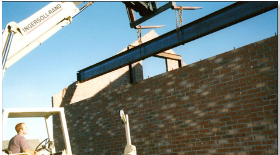
Erection of longitudinal beam.
