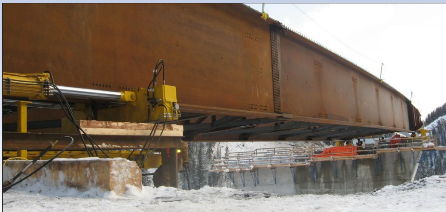
Hydraulic jacks pushing the girder frames.
