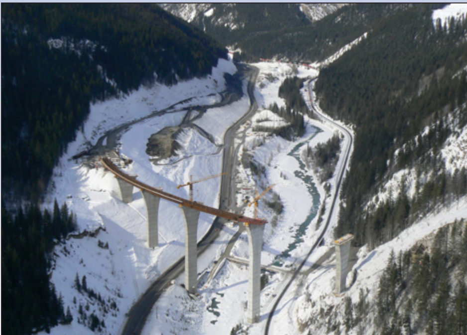
Girder frame crossing the fourth pier.
