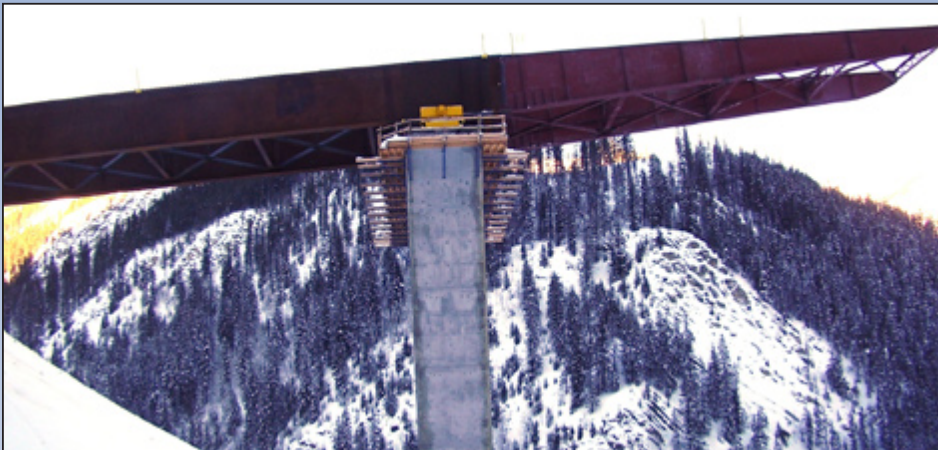
The nose section crosses the first pier.
